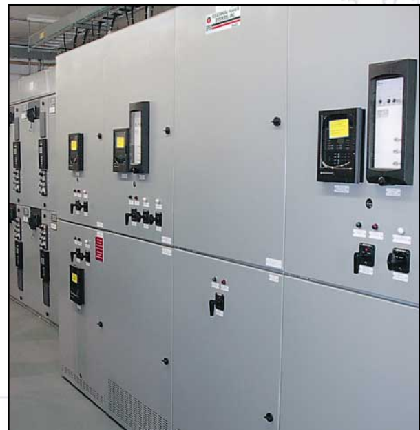
Equipment Installed, Interconnected and Tested in Controlled Factory Conditions by Trained Technicians
