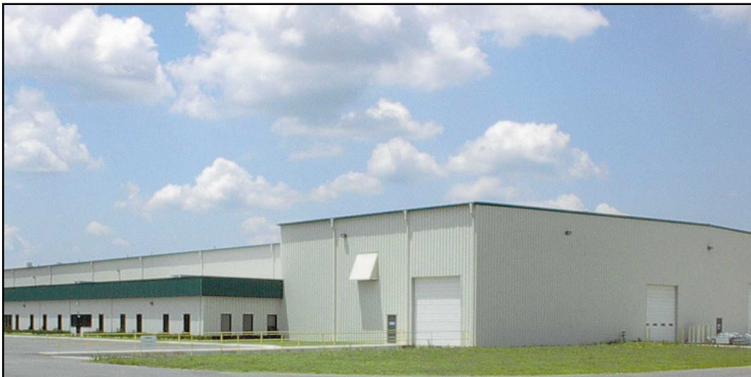
Electrical Power Systems, Inc. 9490 Ridgeway • Tulsa, OK 74131 Phone 918.224.7699 • Fax 918.224.1208
