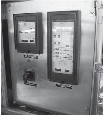
BE1-951 replacing GE-IAC (left) and WH/ABB-CO (right), Nashville, Tennessee
