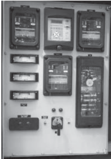
BE1-951 replacing GE-IAC (left) and WH/ABB-CO (right), Nashville, Tennessee
