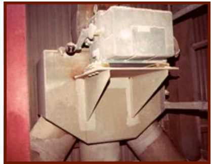
A Jordan SM-5000 electric actuator used in a coal diverter application.
