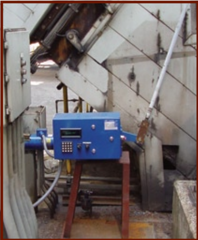
A Jordan SM6000 electric actuator provides continuous modulating duty and 0.1% accuracy for precise damper control.
