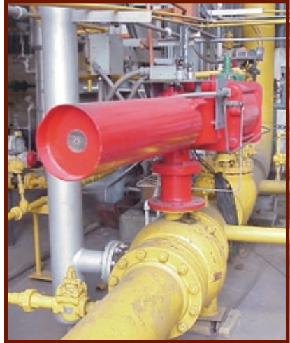
A Rotork Fluid System P-Range spring-return pneumatic actuator operates a block valve in gas service.
